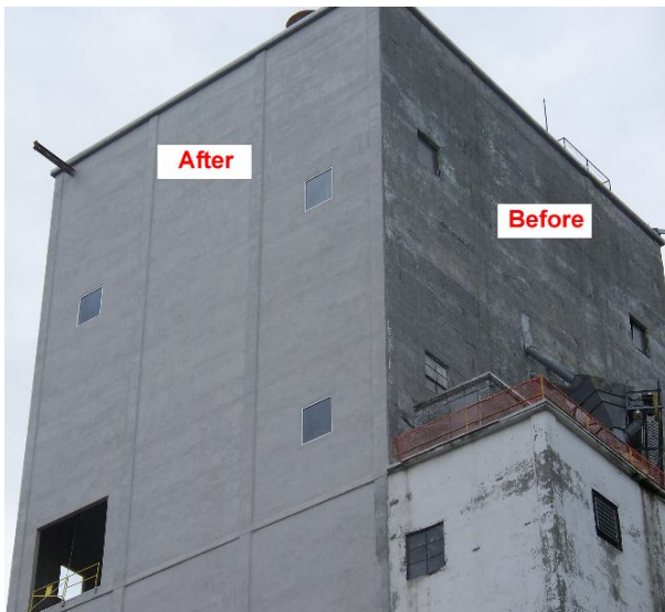
Concrete Repair and Sealing
